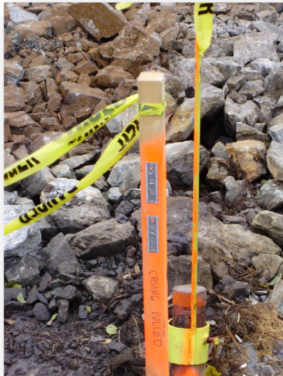
Plate 8 Diamond Drill Casing, Capped and Labeled
