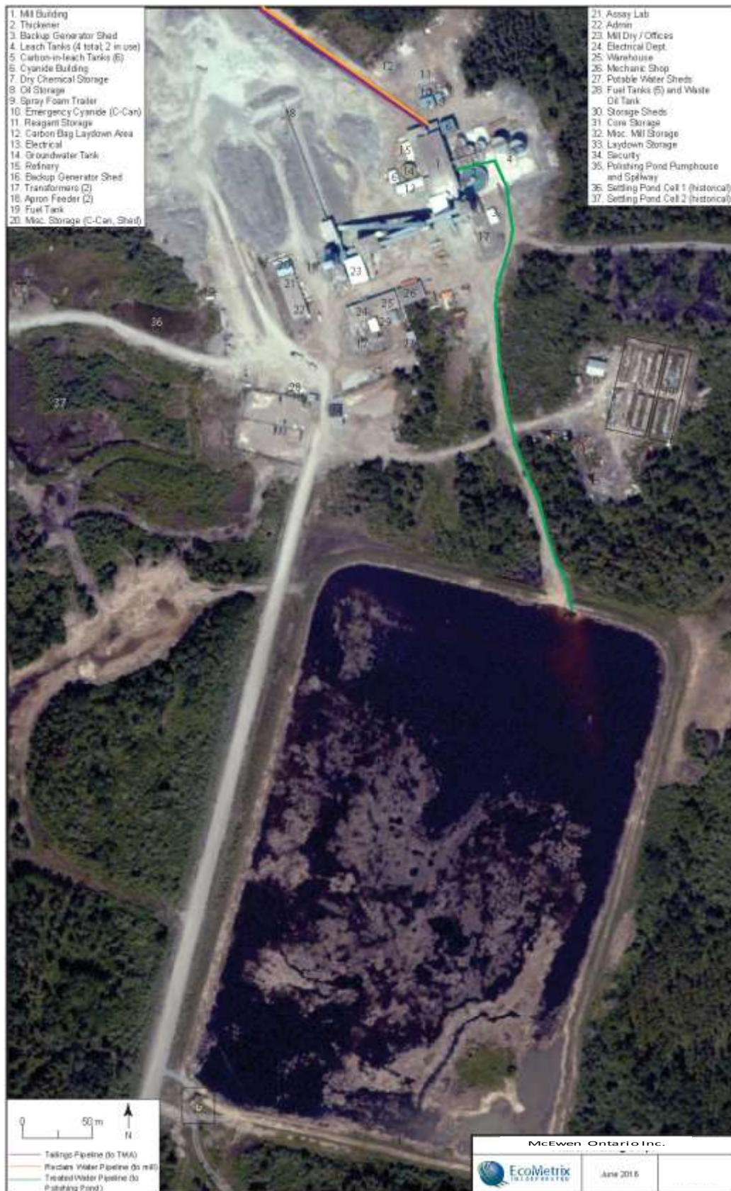
Figure 85: Aerial Image - Black Fox Mill Showing Key Site Infrastructure
