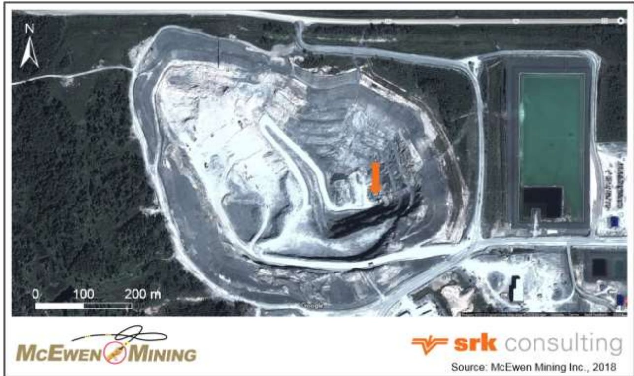
Figure 72: Current Closed Open Pit Houses the Access Portal to Underground Black Fox Mine
