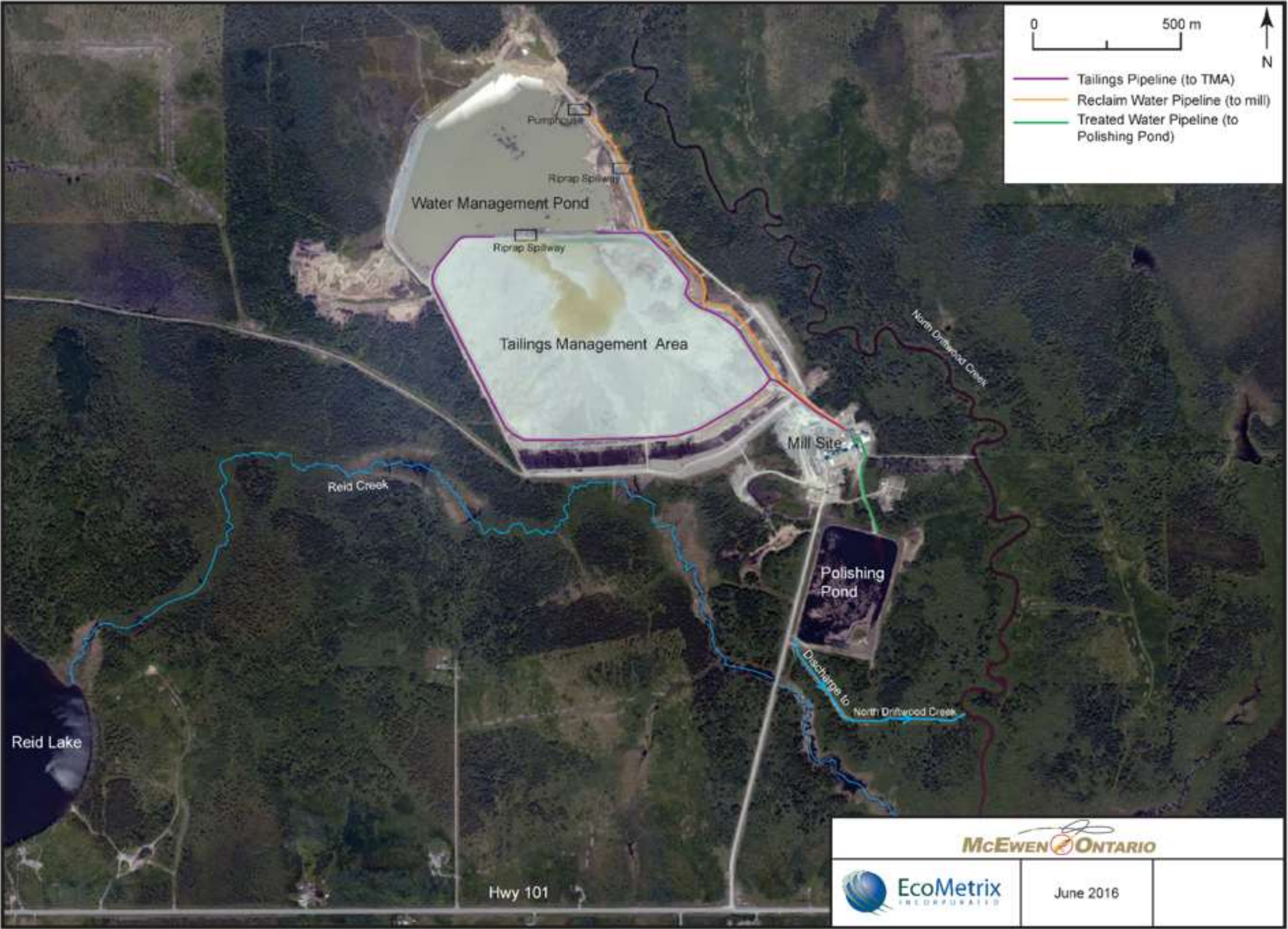
Figure 84: Aerial Image of the Black Fox Mill Showing Major Site Infrastructure and Features of Adjacent Lands
