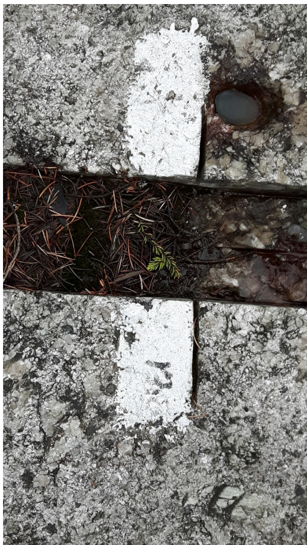
Figure 12-10 Channel SC-01 and a plugger hole on North Dyke
