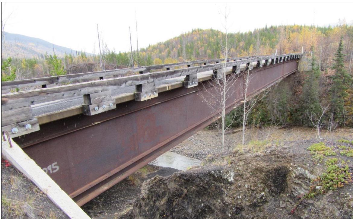
Figure 5.8 The Steel I Beams of Little Iskut Bridge (looking approximately north), Spectrum-GJ Project Area (supplied by the Company)
