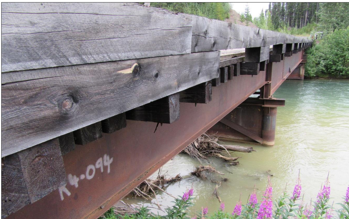
Figure 5.6 The Steel I Beams of Iskut Bridge (looking north-northwest), Spectrum-GJ Project Area (supplied by the Company)
