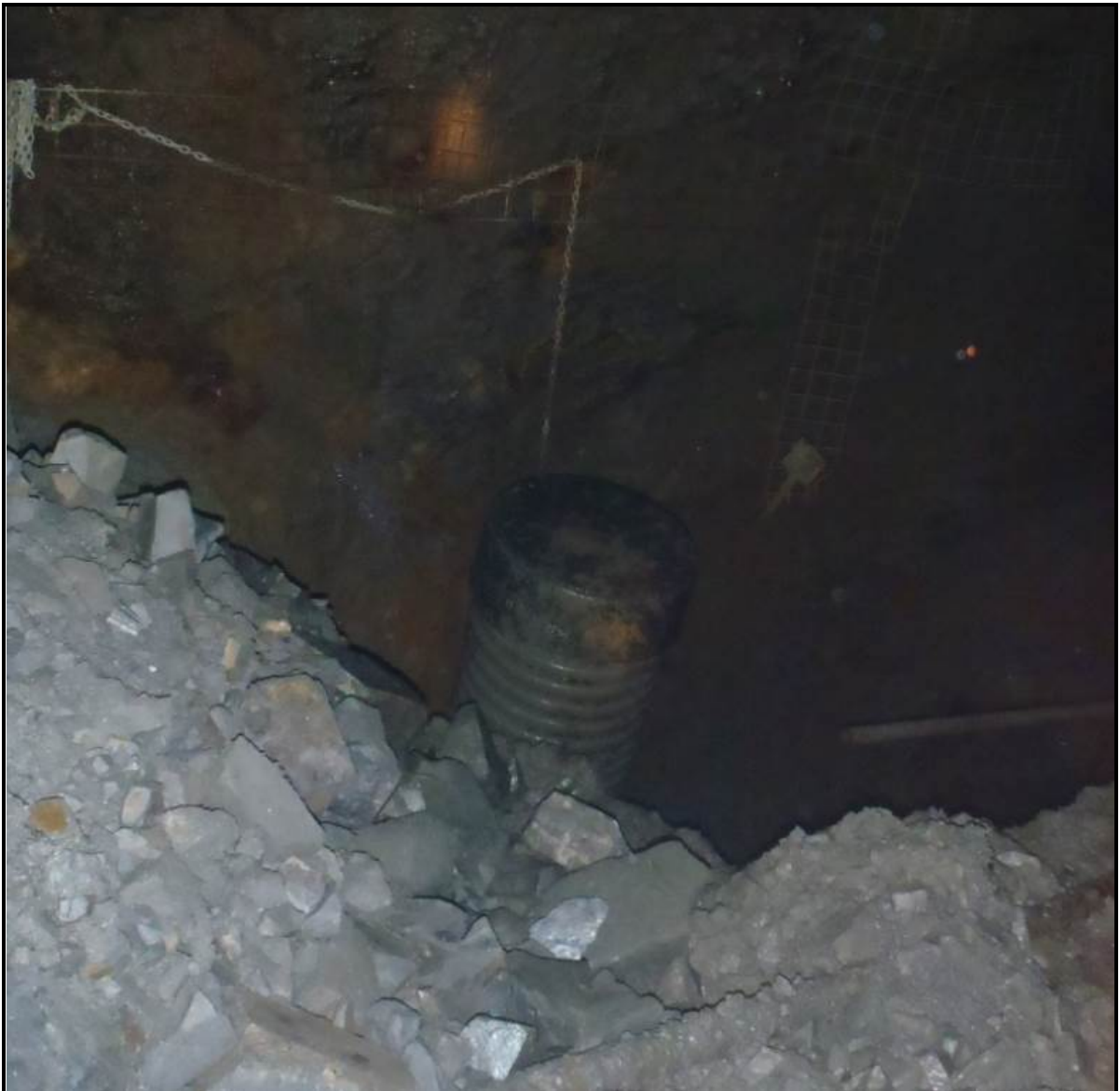
Figure 16.13: Culvert Installed in Longhole Stope (SRK, 2013)
